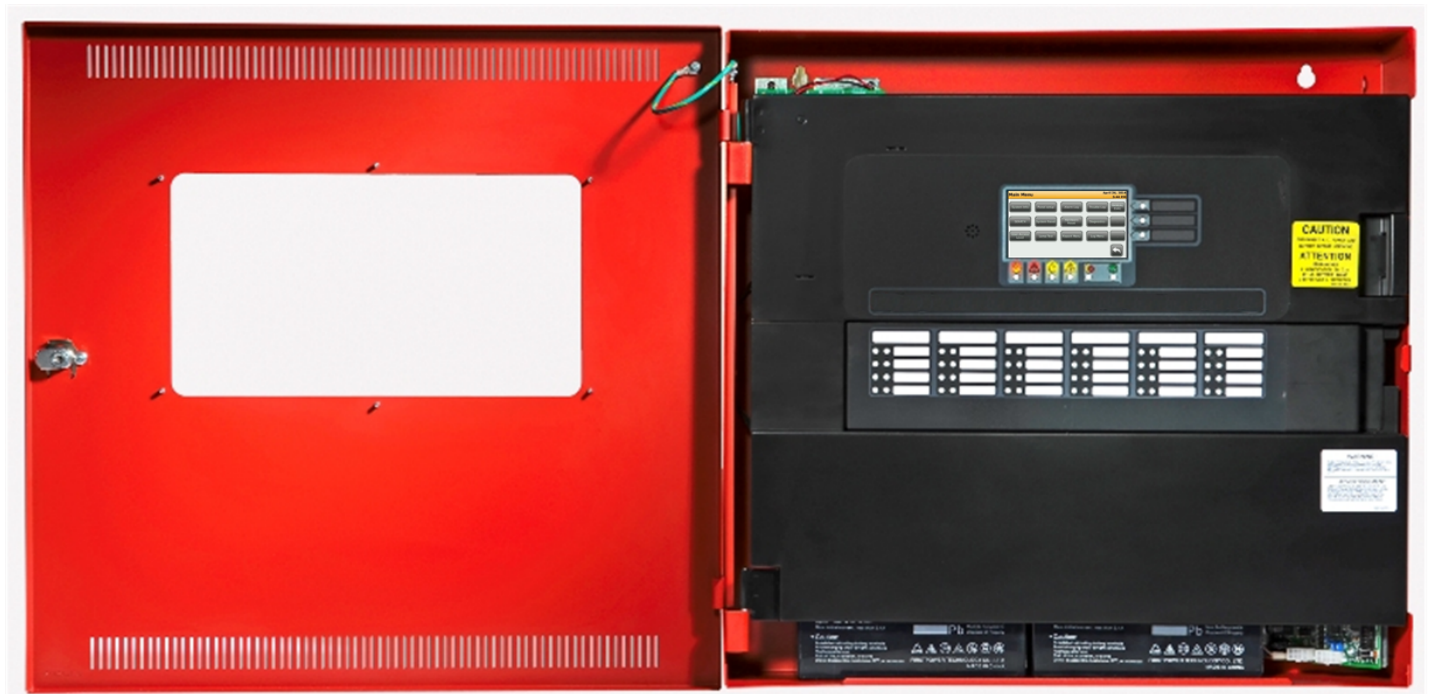
Fig 8: 4007ES Hybrid Operator View with door open
